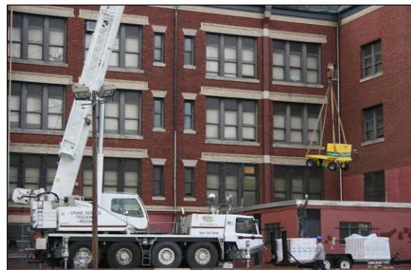
Emergent roofing work progresses at the Avon School in Newark.
