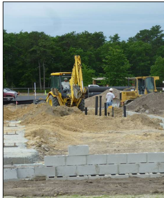
Construction site of the new gymnasium at Reeds Road Elementary School.
