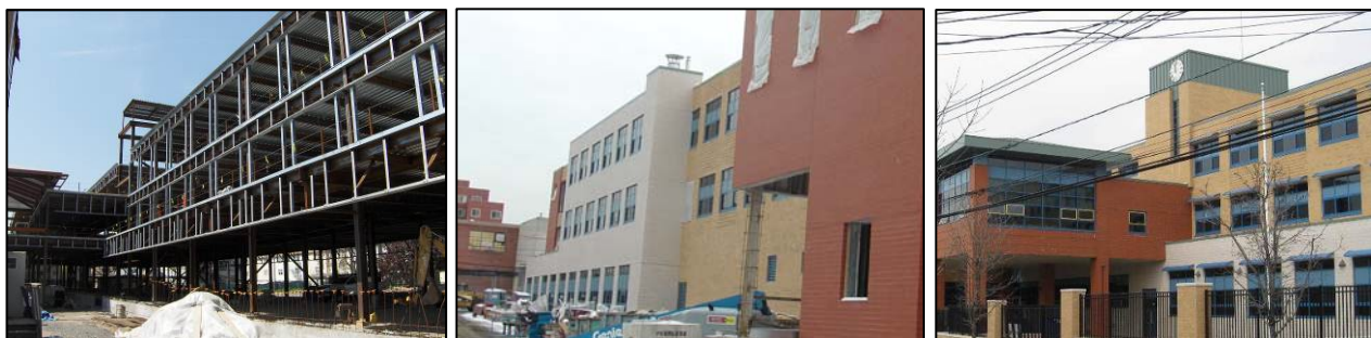
Construction of Public School Number 3 in West New York
