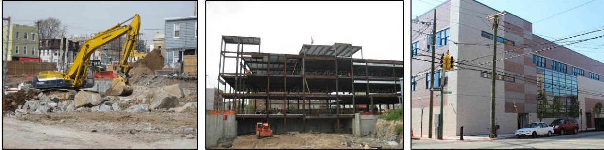
Construction of Colin Powell Elementary School in Union City
