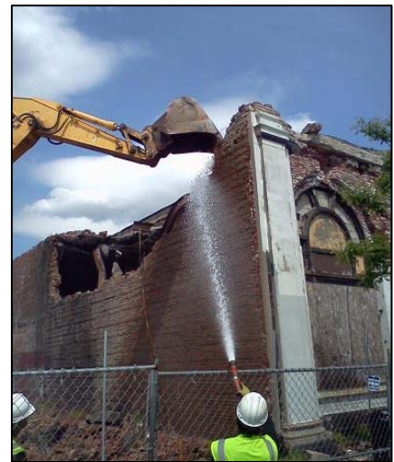
Demolition activities in Jersey City.
