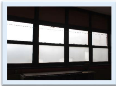
Original windows that were opaque and therefore did not provide appropriate daylight.
