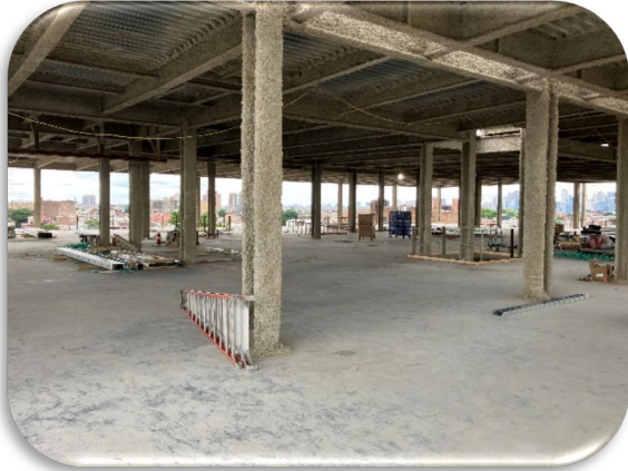
Construction progress of the new Grade 7-9 School in Union City.
